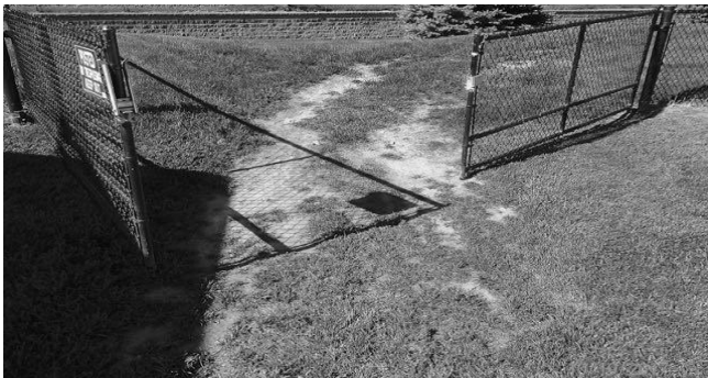
Figure #6 – Spillway Erosion – South Pond
