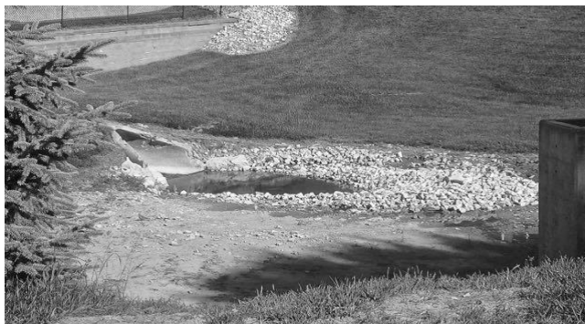
Figure #4 – South Pond – Erosion/Standing Water
