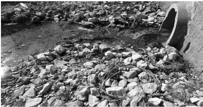
Figure #5 – North Pond – Destroyed Wire Cage
