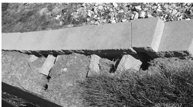
Figure #1 - North Detention Pond – West Wall Erosion
