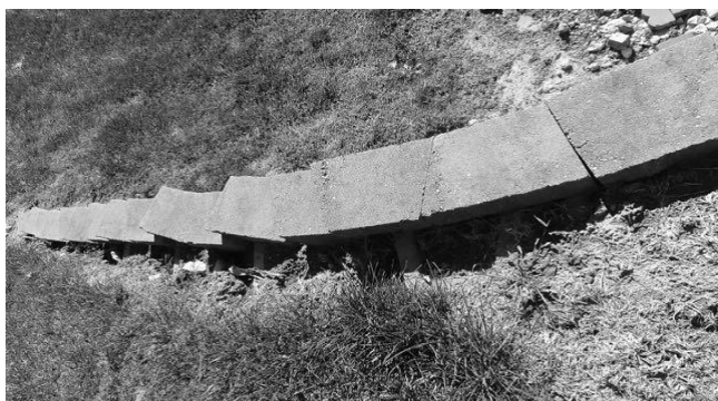
Figure #2 - North Detention Pond – West Wall Erosion
