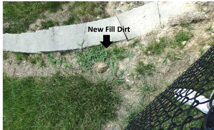
Figure #5 – Example of new fill behind stone wall
