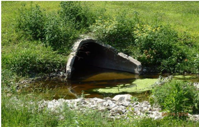
Figure #1 - Scour Hole & Destroyed Wire Baskets – July 2014
