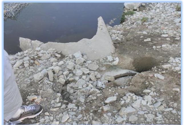
Figure 3 - South Pond 7/8/14 – Eroded Inlet Pipe
