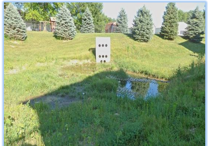
Figure 5 - South Pond July 2019 Grass & Weed Control Challenging
