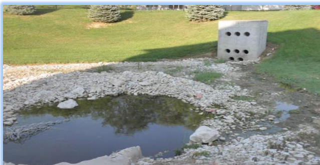
Figure 2- South Pond 7/8/14 Scour Hole - Empty Basket
